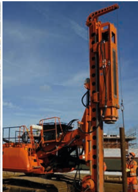
DX RIG MOUNTED DRIVING TUBES
